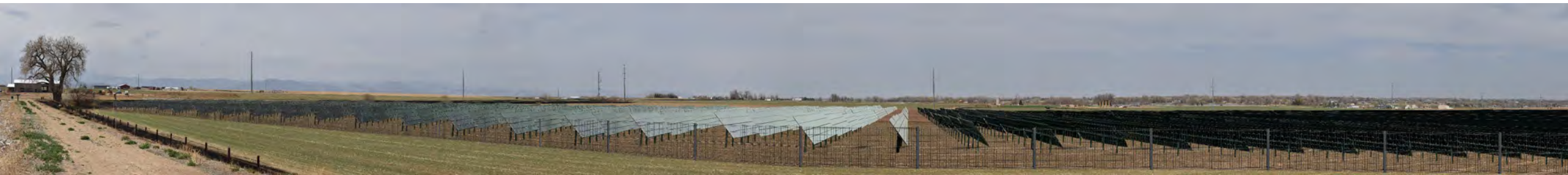
Solar Panel Installation *Screening not shown but would be included per Town standards along the right-of-way
