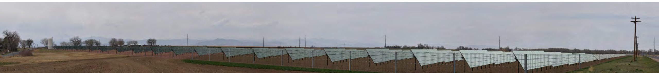
Solar Panel Installation *Screening not shown but would be included per Town standards along the right-of-way
