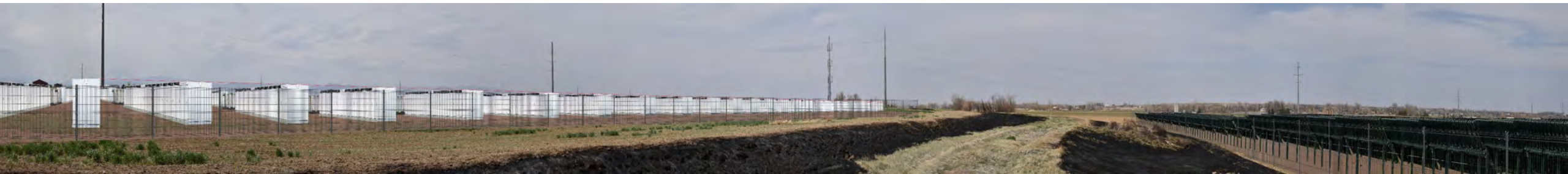
Battery Energy Storage and Solar Installation
