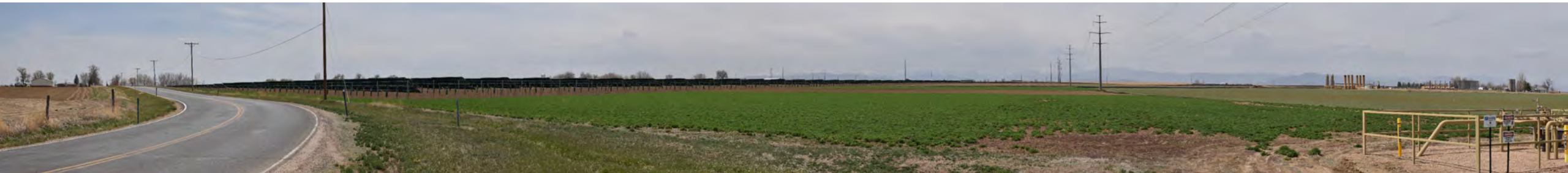
Solar Panel Installation *Screening not shown but would be included per Town standards along the right-of-way
