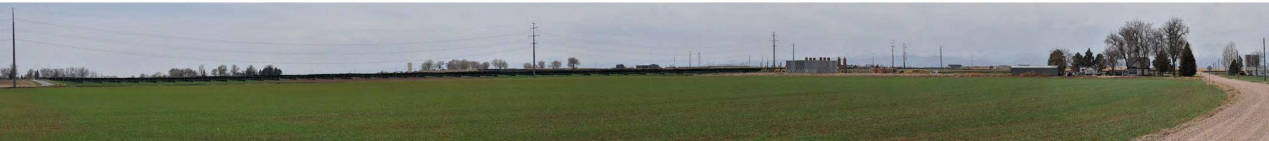
Solar Panel Installation *Screening not shown but would be included per Town standards along the right-of-way
