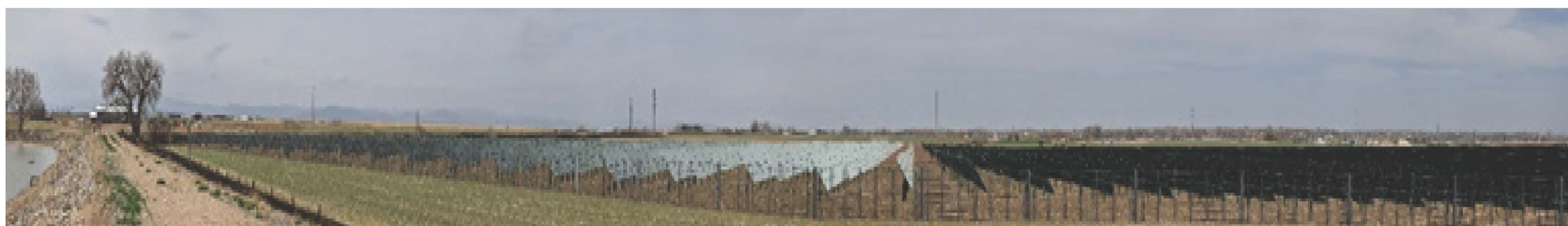
5- Solar Arrays as Looking East from Town of Mead Reservoir.
