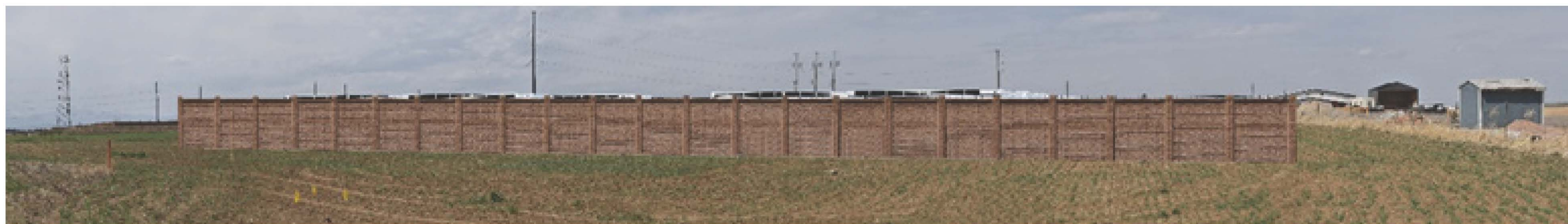
2- Potential Screening with Block Wall, which could replace the Ornamental Metal Fence to match the Longs Peak Substation seen at left.
